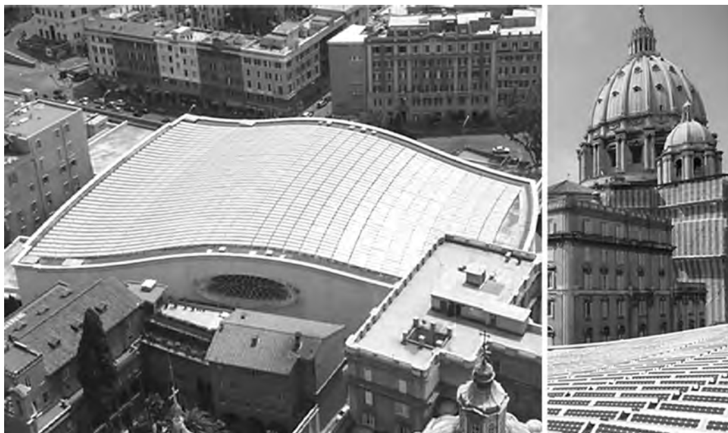
Fig. 4. Photovoltaic system integrated on the roof of Aula Pierluigi Nervi, Vatican.
